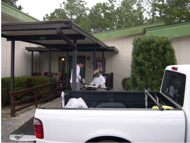
Horizons' maintenance staff adding yet another countertop for additional space.
