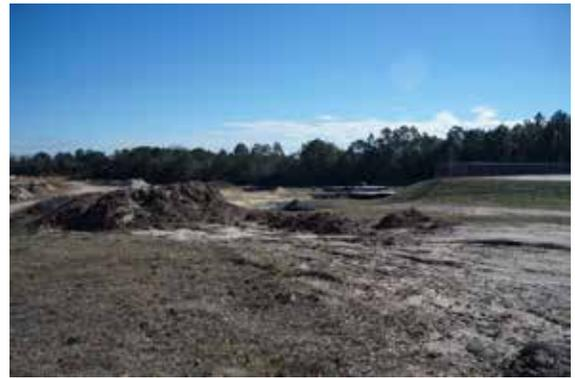
Photographs looking west show refuse stored on site and the slopes of the fill used to raise the Public Safety building to street level at 220 feet elevation.
